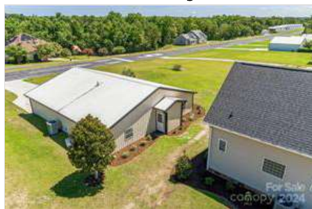
Aerial Hangar & House
