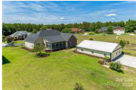
Aerial House & Hangar
